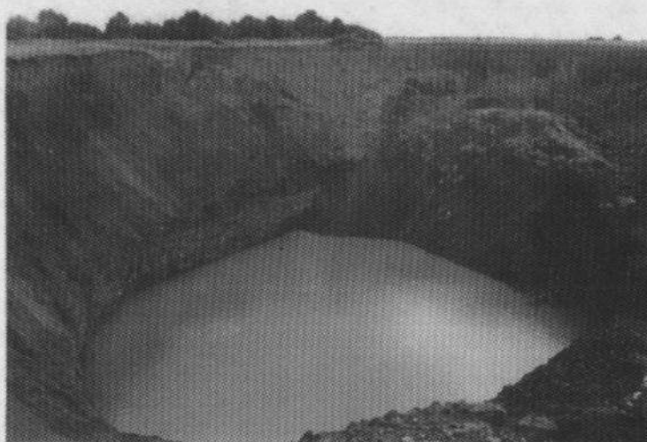
Figure 16. Collapse caused by SG4-SG5 cavities at Gellenoncourt in 1998 (CSME & École des Mines de Paris document)
