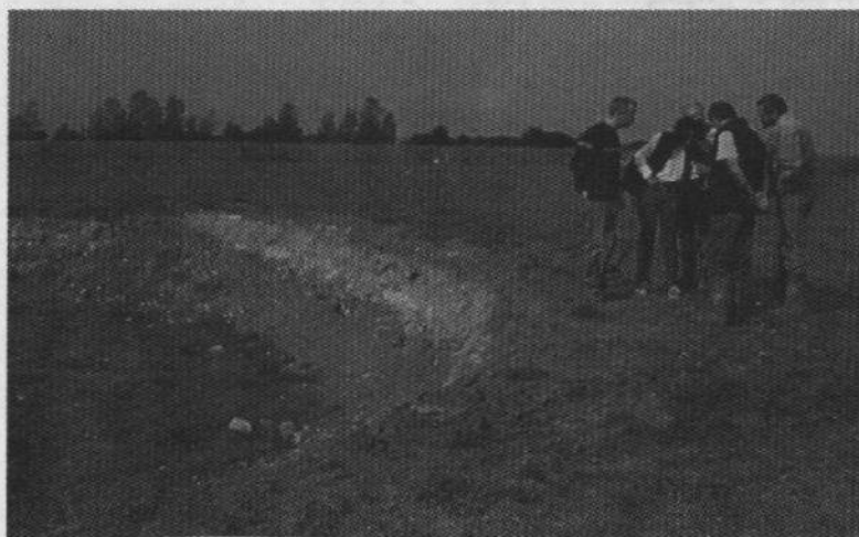
Figure 3. Settling of backfill of a crater created by the collapse of a solution mining cavern. Nancy basin
